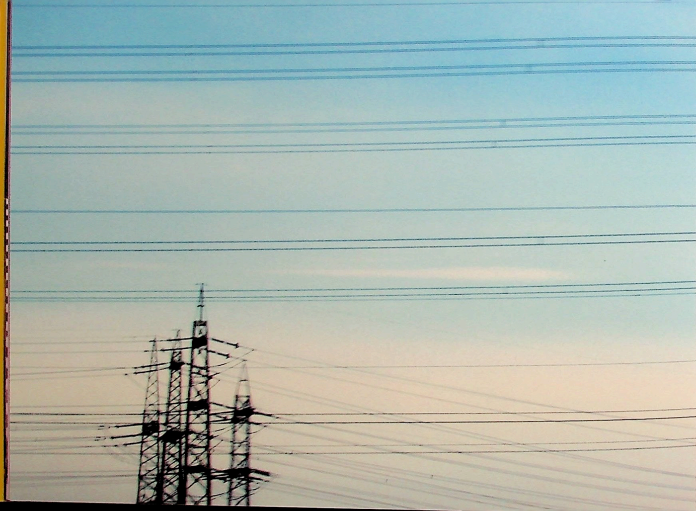
Wires on the highway / Lignes hautes - tension
